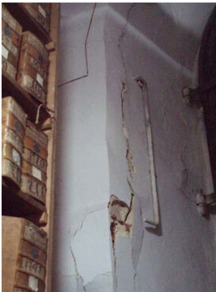
Cracked walls let in moisture and humidity that are harmful to the Archives' records
